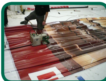
Track Welding on Floor
